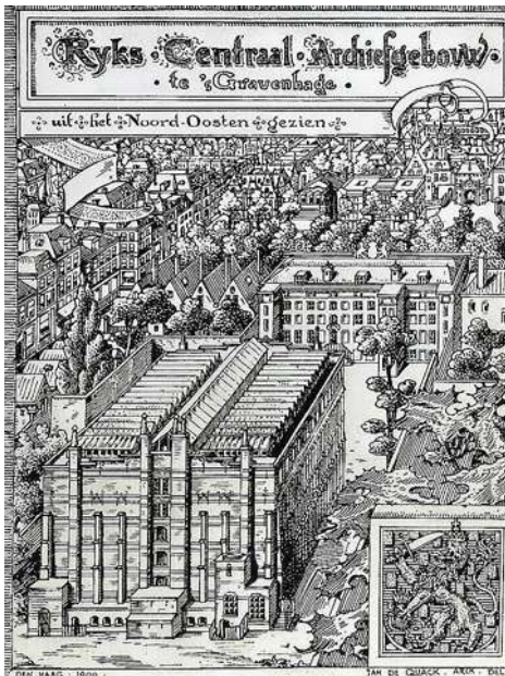
Fig. 11.18a The repository of the National Archives ( Rijksarchief ) in The Hague, built in 1899. Drawing by Jan de Quack, 1900. In 1902 the office building of the Rijksarchief was built in front of the repository.
